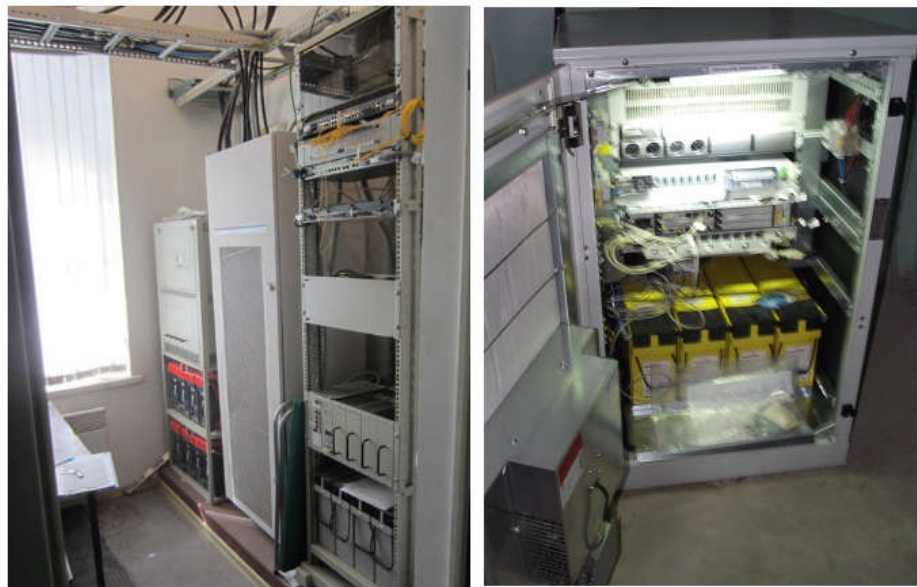
Figure 4 Deep edge hosting environment, based on a typical RAN site layout
